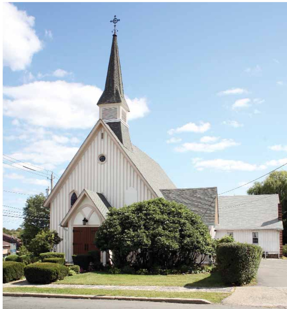
St. Paul's, Spring Valley. Grants from Property Support and the Bedell Fund funded structural repairs as well as the painting of the church exterior in historically appropriate colors.
